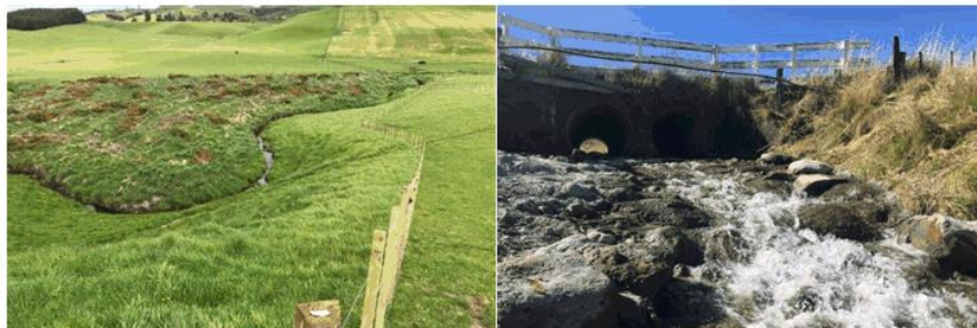
Photo 6 and Photo 7 Fencing and fish pass work completed in the Whangaehu Catchment under the Freshwater Improvement Fund project.
